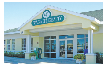
5215 SR 64 East Bradenton, Florida
